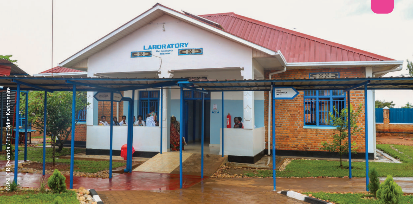
A health center in Mahama Refugee Camp
