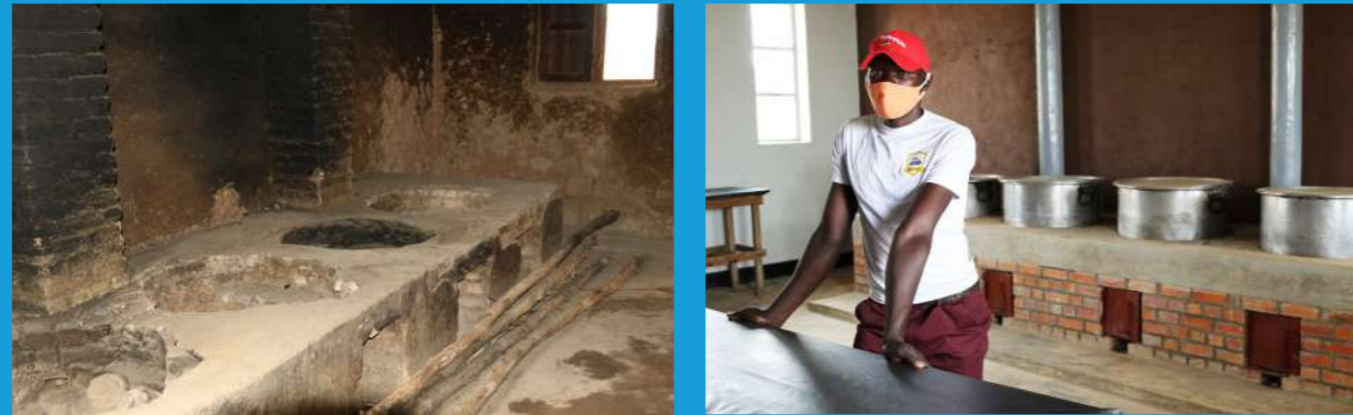
The contrast between old (left) and new (right) kitchen is stark. School cook Felicien Rwatangaro is pleased with the new facilities and looks forward to welcoming students back.
